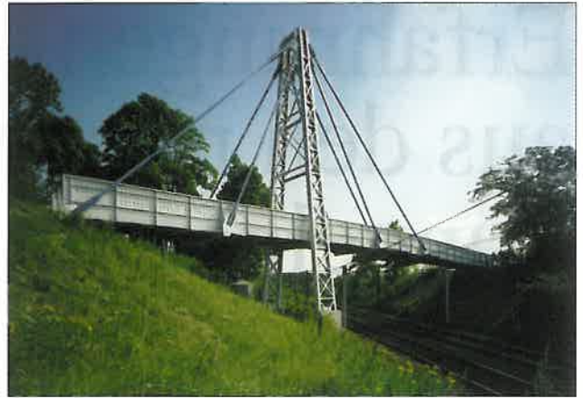
Abb. 11: Fiberlinebrücke in Kolding (System: Fiberline)
