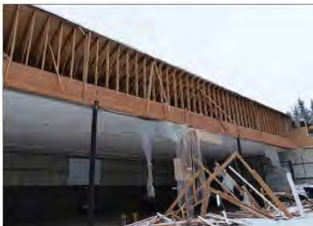
Fig. 1: Remaining roof structure from case study 1
