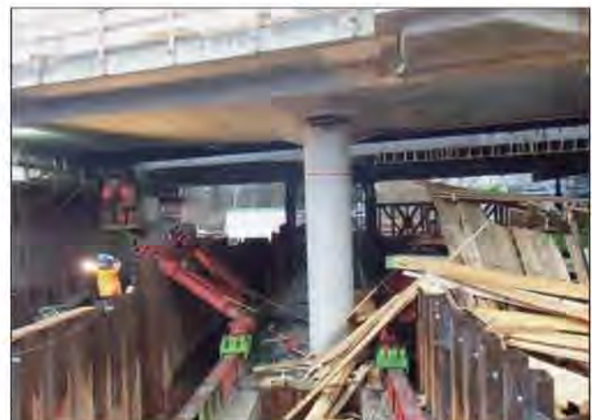
Fig. 2: Debris of formwork from case study 2
