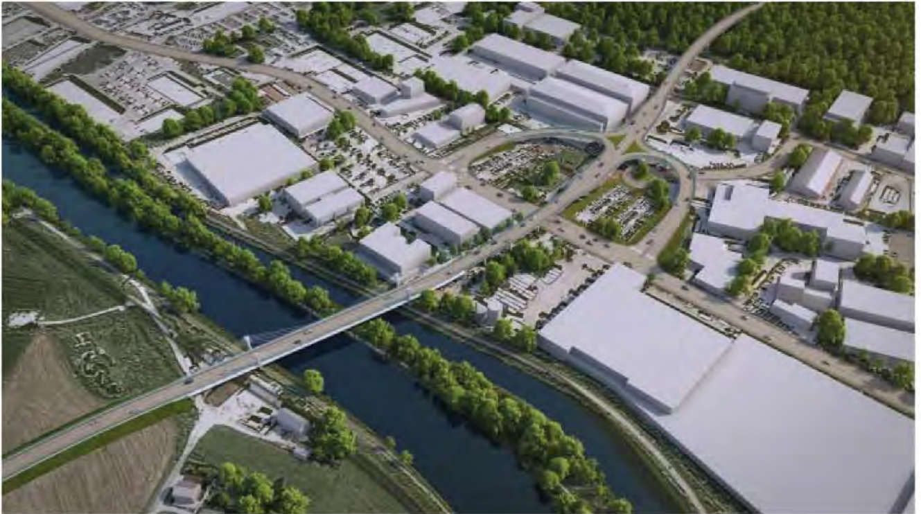
Figure 2. Extradosed and multi-span composite bridges ©OVB
